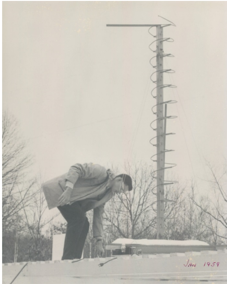
January 1959, with 400-MHz antenna
