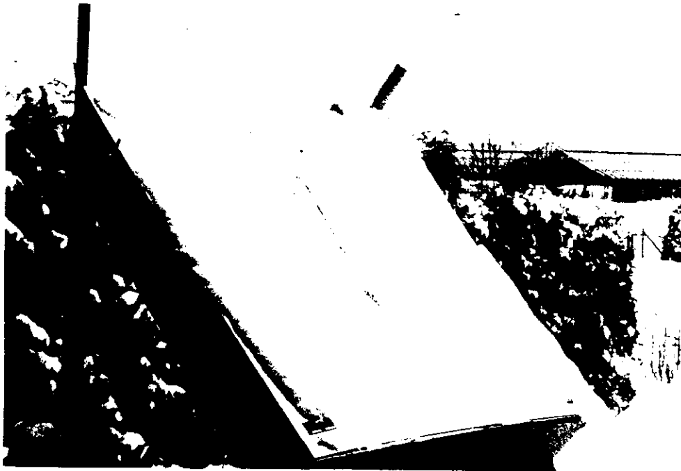
DEICING SYSTEM NATURAL TEST
