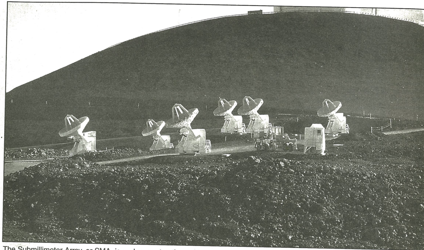
The Submillimeter Array, or SMA, is under construction on Mauna Kea and is expected to be completed by November.
